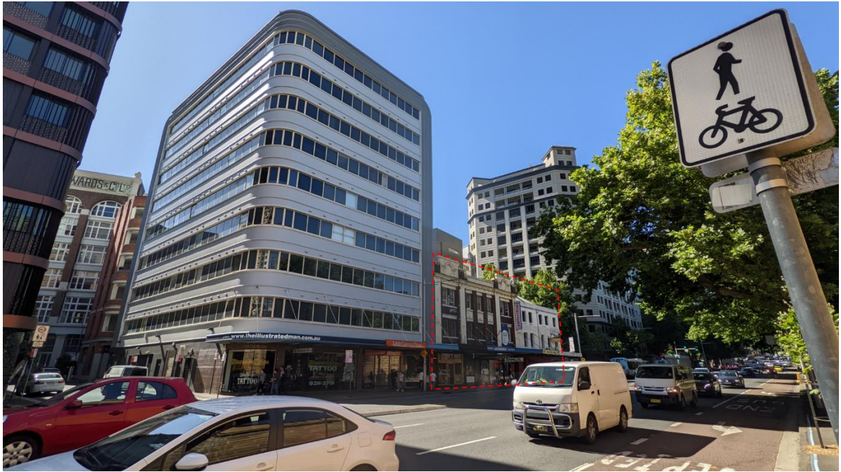
Figure 3 - The site viewed looking south east along Elizabeth Street
